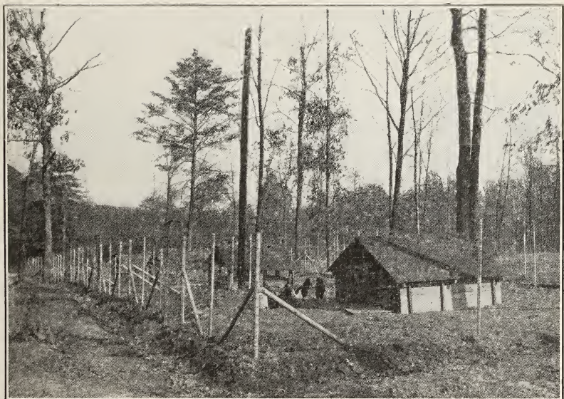
FIGURE 25.—Experimental pens for fowls used in parasite investigations. The wire fencing is stretched on steel posts set in concrete. A 5-foot lane is provided between the pens to keep the birds of the different pens from having any contact through the fence. The semiopen shelters are equipped with wire floors to prevent the birds from having access to droppings.
